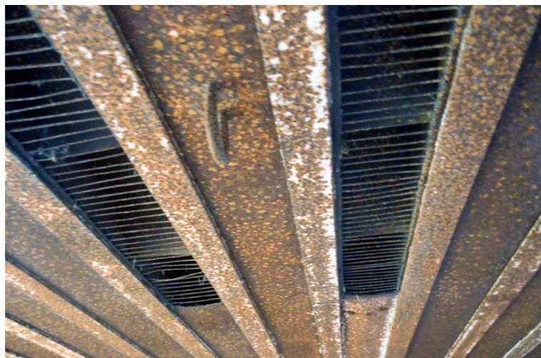
**Figure 9.** Kullak battery : R669 (b)—fire room ceiling, grids of the combat gas extraction system and one of the two joints for the gun lifting.
