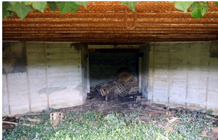
**Figure 8.** Kullak battery: R669 (b) fire room—at the centre walled rear side aperture, on the left entrance of the ammunition room, on the right entrance of the combat gas extraction system room, on the metal ceiling two joints for the gun lifting, on the left and right walls panels of the thermal or acoustic insulation system.
