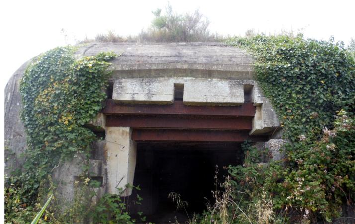
**Figure 11.** Kullak battery: R669 (c) front side aperture of the fire room with splinter guards partially covered by the vegetation.
