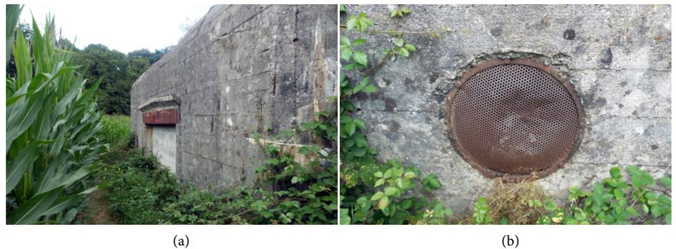
**Figure 12.** Kullak battery: (a) R669 (c)—walled rear side aperture; (b) R669 (c)—grid on the exhausted combat gas pipe.
