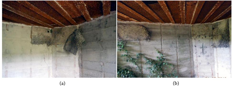
**Figure 7.** Kullak battery: (a), (b) R669 (b) interior of the fire room with panels of the thermal and/or acoustic insulation system on the walls.
