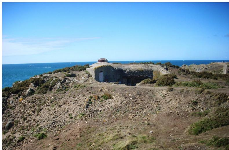
**Figure 16.** Pointe de la Varde support point: R120a observatory bunker ( $48^{\circ}40'53.4''\text{N}$ ,  $1^{\circ}59'23.4''\text{W}$ )—on the left, white painted, entrance of the uncovered lookout post and the observatory bell, in the middle bunker entrance and close combat room, on the right protective wing.
