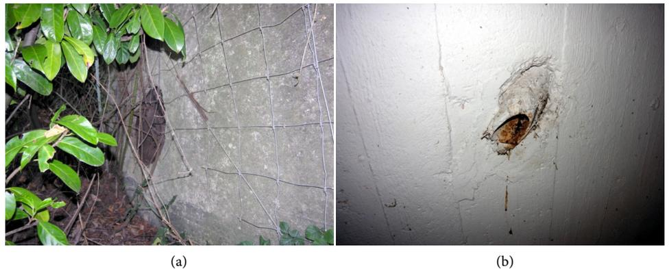
**Figure 28.** Les Ormeaux battery: (a) R669—air vents on the front facade ; (b) R669—cable passage on the front facade.
