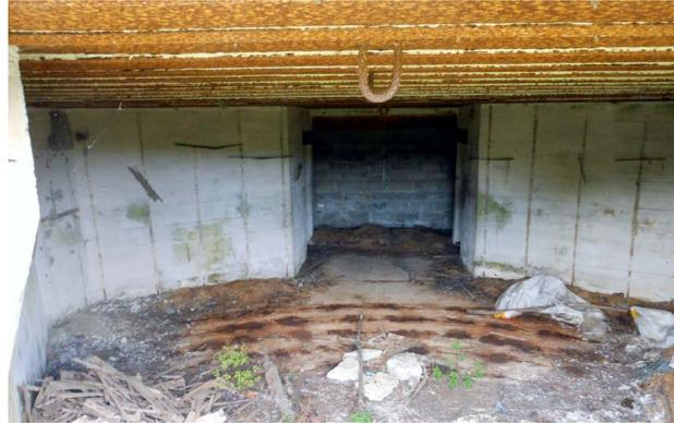
**Figure 13.** Kullak battery: R669 (c) fire room—at the centre walled rear side aperture, on the left entrance of the ammunition room, on the right entrance of the combat gas extraction system room, on the metal ceiling two joints for the gun lifting, on the floor arcuate rails of the vibration dampening system, on the left and on the right wall rests of the supports for the panels of the thermal and/or acoustic insulation system, on the floor arcuate rails of the vibration dampening system.
