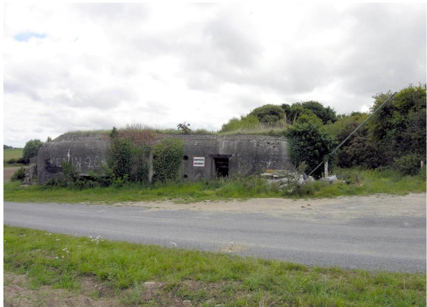
**Figure 22.** Ville Besnard logistic base: lonely bunker—on the left front aperture of the fire room, at the road level, on the centre four air vents, on the right personnel entrance, behind the bunker, cistern area (a2).
