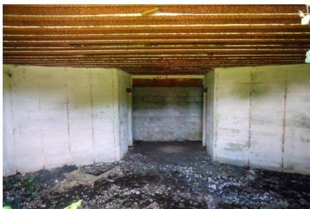
**Figure 5.** Kullak battery: R669 (a) fire room—at the centre walled rear side aperture, on the left entrance of the ammunition room, on the right entrance of the combat gas extraction system room, on the metal ceiling distorted joint for the gun lifting.
