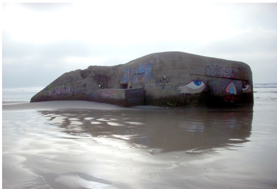
Figure 20. Wn. Qu. 39—details of the H501: on the left protection wing with opening of the tobruck for machine gun, at the center entrance with protective wall.
