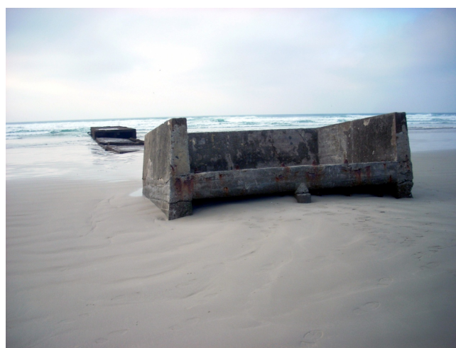
Figure 15. Aqueduct component (3) with the possible location of the opening and closing mechanism of the doors with protective wall, on the left component (1) and between the two, the component (2) covered by sand.
