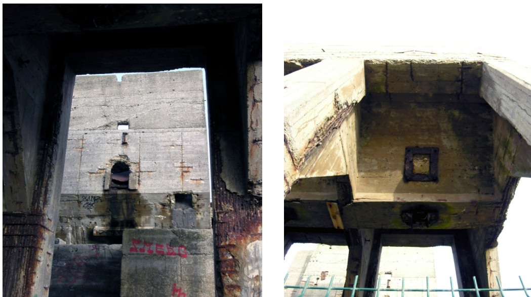
Figure 31. Todt Camp—release door for the crushed pebbles of the second crusher compartment and release doors for the crushed pebbles of the first silo for charging the crushed pebbles on wagons.
