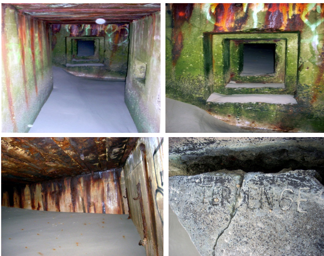
Figure 21. Wn. Qu. 39—details of the inside of the H501—access corridor with embrasure, bunk beds supports for the troop, engraved in scripton or TER (?) ENGE or TER (?) EN6E.
