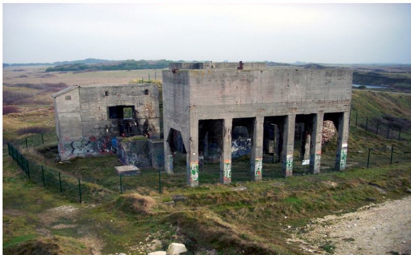
Figure 28. Camp Todt—remains of the crusher building, on the left electric distribution cabin and first crusher compartment, in the middle the first silo for crushed pebbles.
