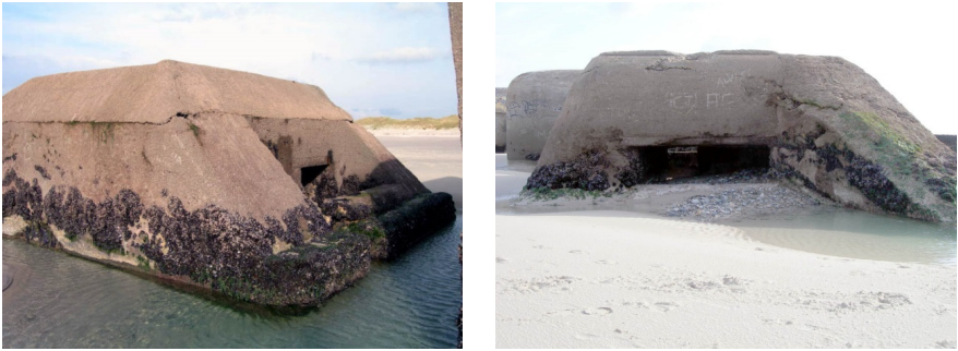
Figure 19. Wn. Qu. 39—details of the H667-entrance and embrasure of the firing chamber with protective wing.
