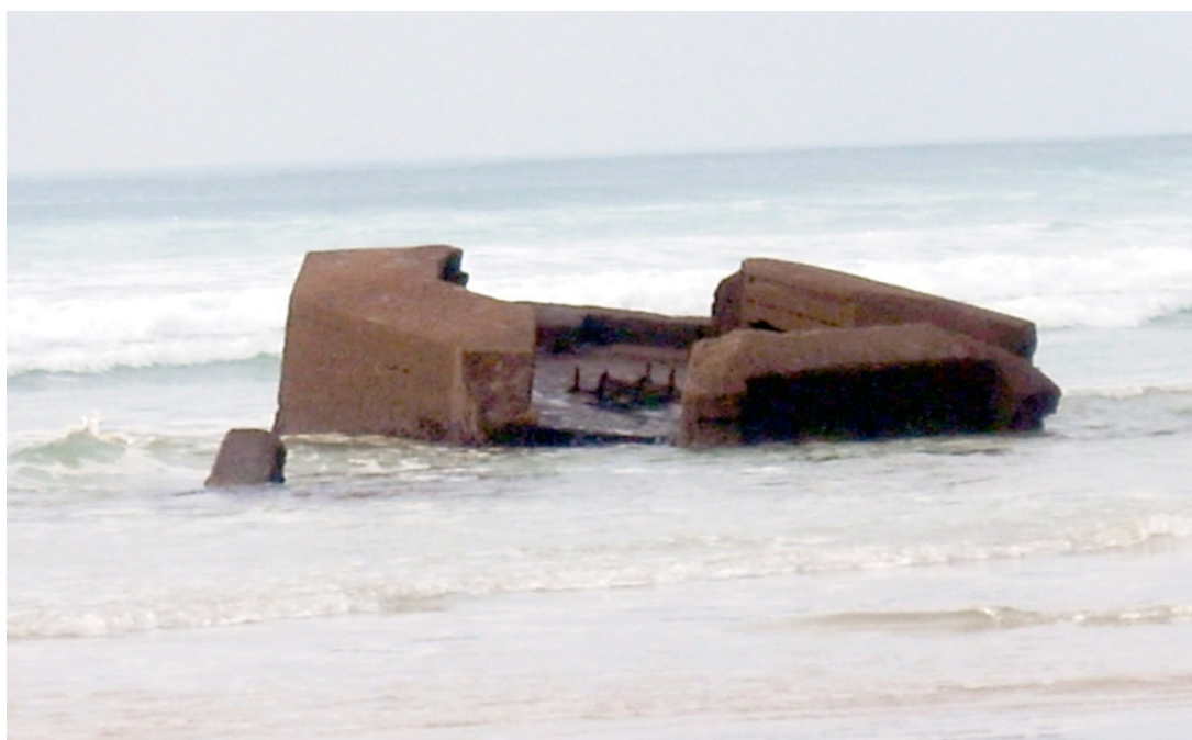
Figure 23. Wn. Qu. 39—Vf600v visible are the mounting studs for the gun 5 cm KwK39.
