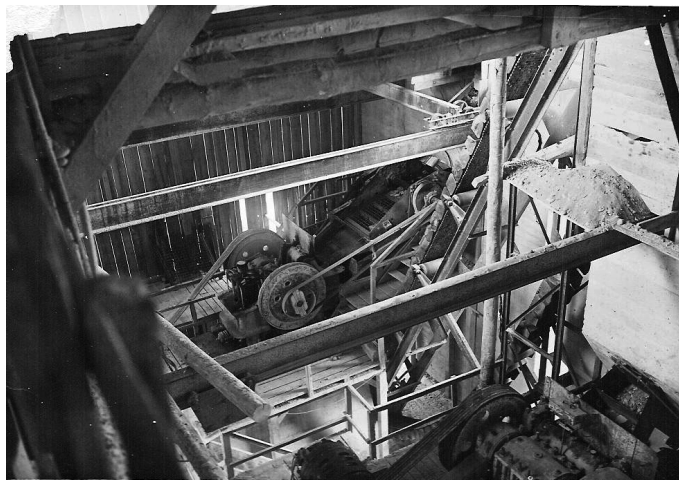
Figure 6. Interior of the crusher building-loading mechanism of crushed pebbles in the first concrete silo.
