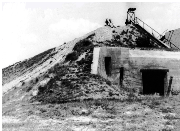
Figure 7. Wn. Qu. 40—bunker H672 of Wn. Qu. 40 at the end of the massive wall, on the left entrance of the tobruck annexed to the bunker, on the right staircase leading straight to the top of the wall and the second silo.
