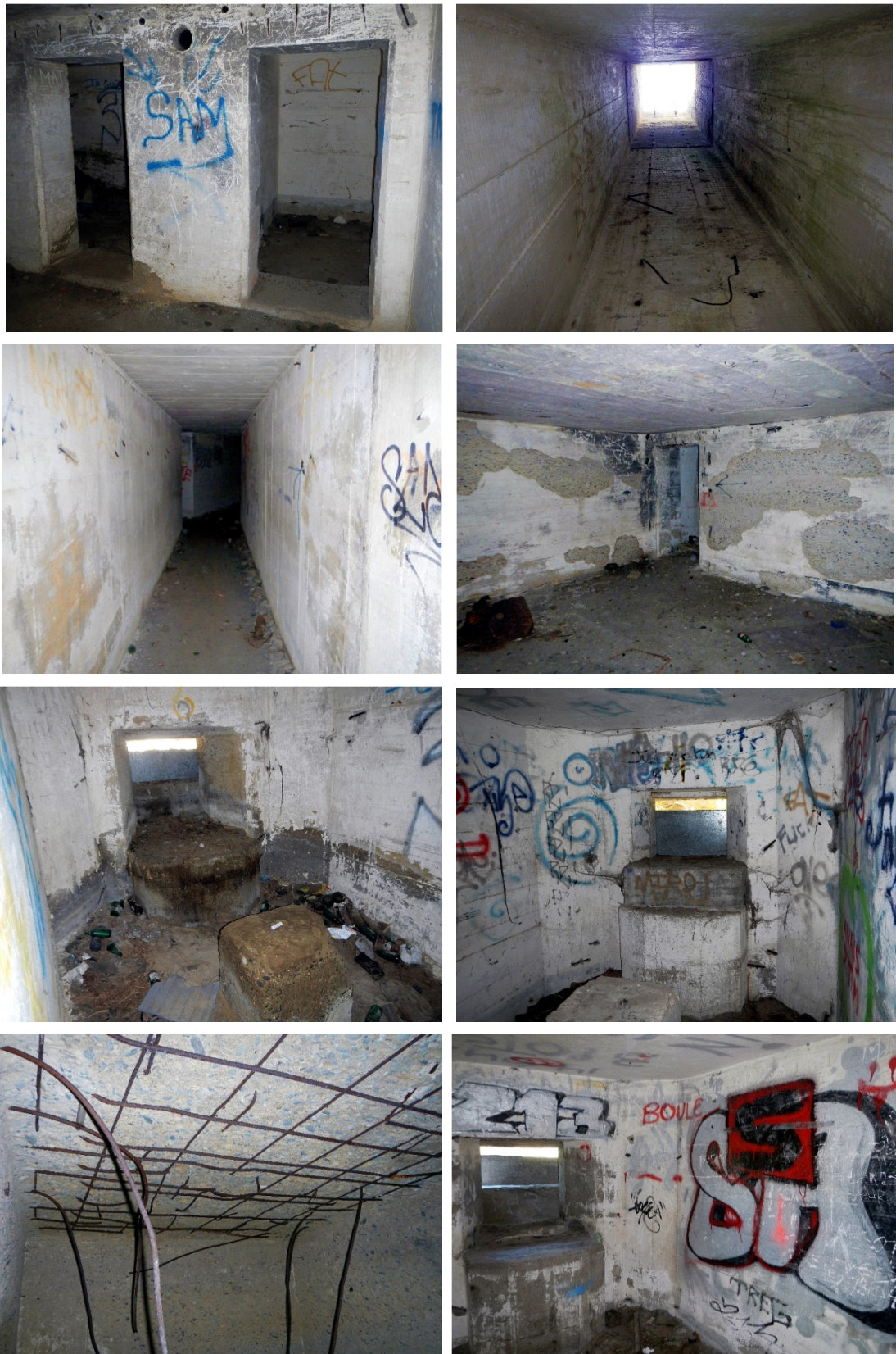
Figure 35. Wn. Qu. 40—details of the connecting passage and the firing chamber sofa Vf bunker.
