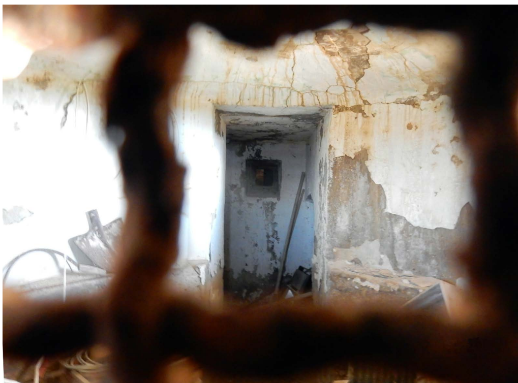
Figure 7. View of the gun chamber, in the middle interior wall with embrasure for the internal defence of the bunker, on the bottom left and right sides portions of the circular shelf.
