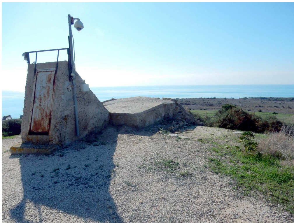
Figure 3. On the left side, inclined entrance portal of the bunker with the original metallic door, a railing and the tele-camera for monitoring the archaeological site, on the right side is visible the top protection of the soldier shelter and the slight arcuate roof of the gun chamber.
