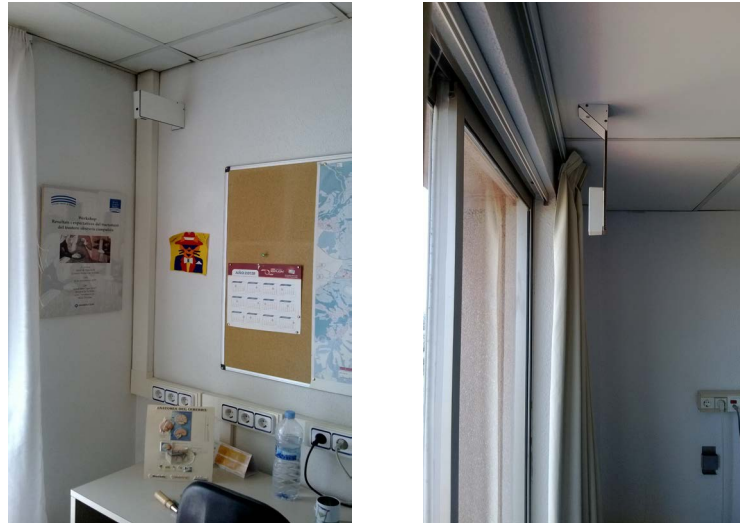
Figure 3. IR wall temperature sensor installation at Terrassa hospital in the case of a wall (side wall mounted) and a window (ceiling mounted) planned for retrofit.
