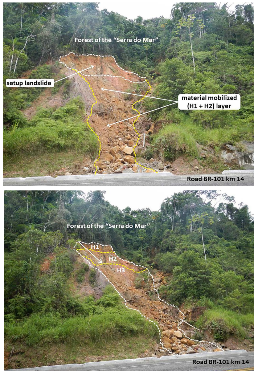
Figure 9. Reactivation of landslide on the slope of Serra do Mar (yellow dot 2 in Figure 10), occurred in Ubatuba between 01/03/2013 and 01/04/2013 in the km 14 of the highway BR-101 (Source: Geological Institute).
