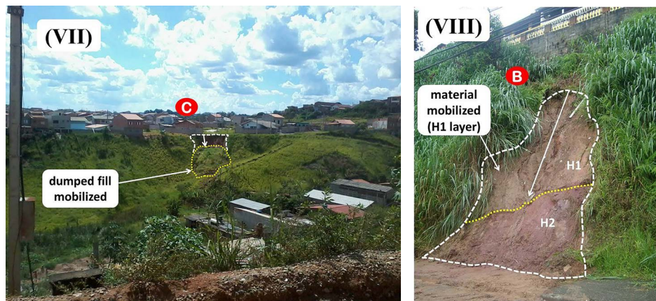
Figure 7. (VII) and (VIII) landslides of the type C (dumped fill) and B, respectively, occurred in São José dos Campos between 01/10/2013 and 01/11/2013 (Sources: VII, authors and VIII, Civil Defense of São José dos Campos).
